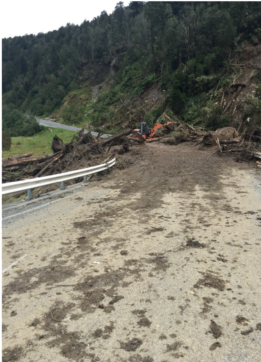
Clearing the road
