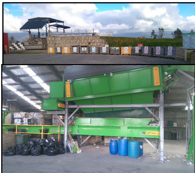
Figure 7: Westport Transfer Station - Drop-off area and MRF
